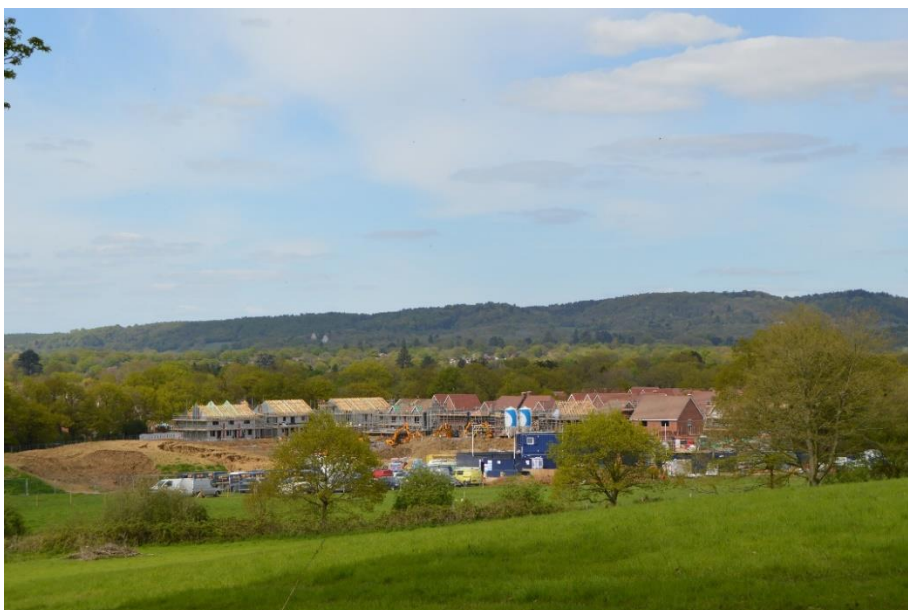
Figure 9: Phase One of development site at Horsham Road under construction
