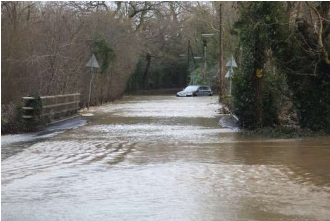
Figure 35: Elmbridge Road Flooding December 2013
