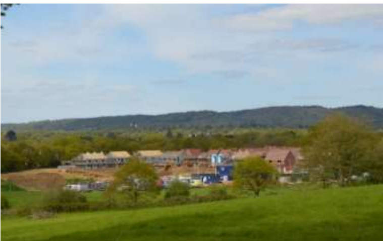
Figure 10: Phase One of development site at Horsham Road under construction
