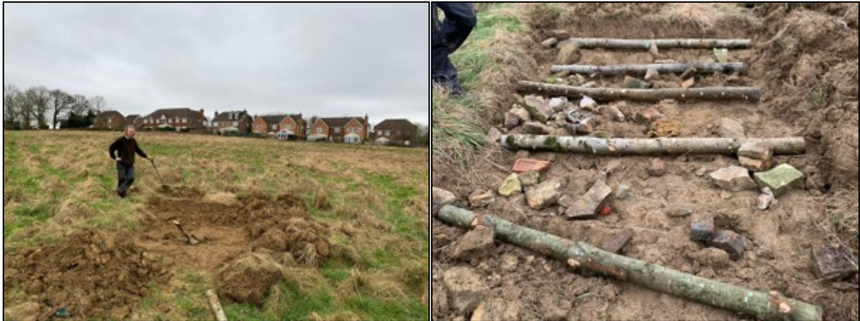
Photo 1a and 1b. Left illustrates the initial digging phase, right illustrates the initial layer of rocks/stone going in.
