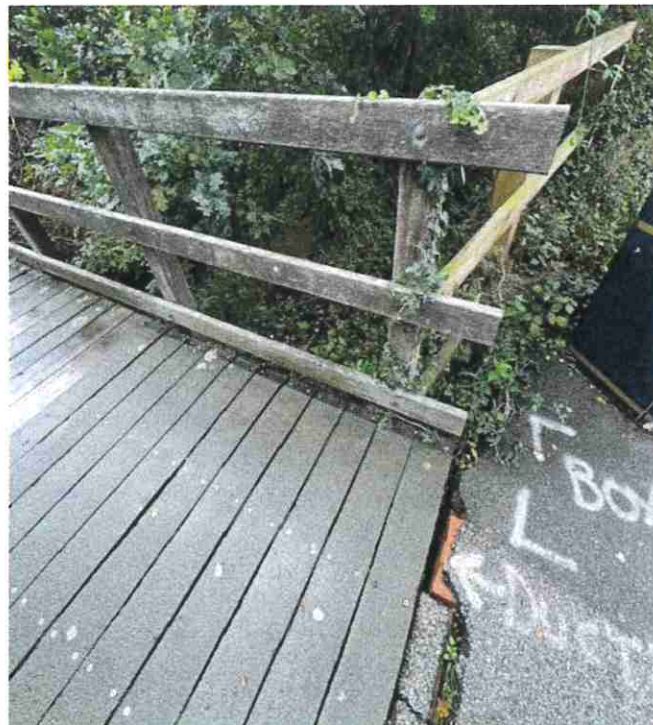
Fig 4: Existing bridge showing the tarmac pavement cracking at abutment with the bridge
