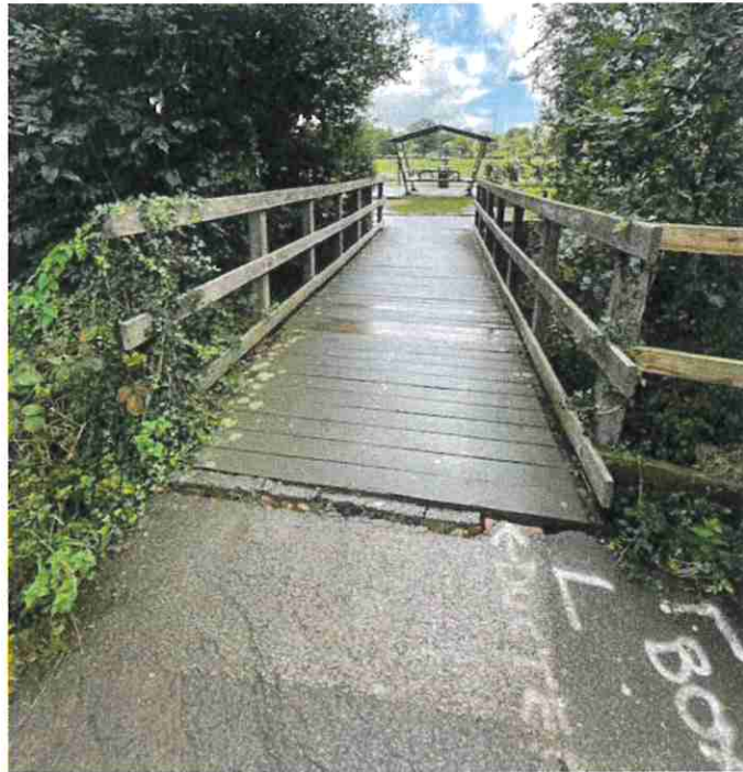
Fig 3: Existing bridge looking south towards the Snoxhall Fields, showing the tarmac pavement cracking at abutment with the bridge
