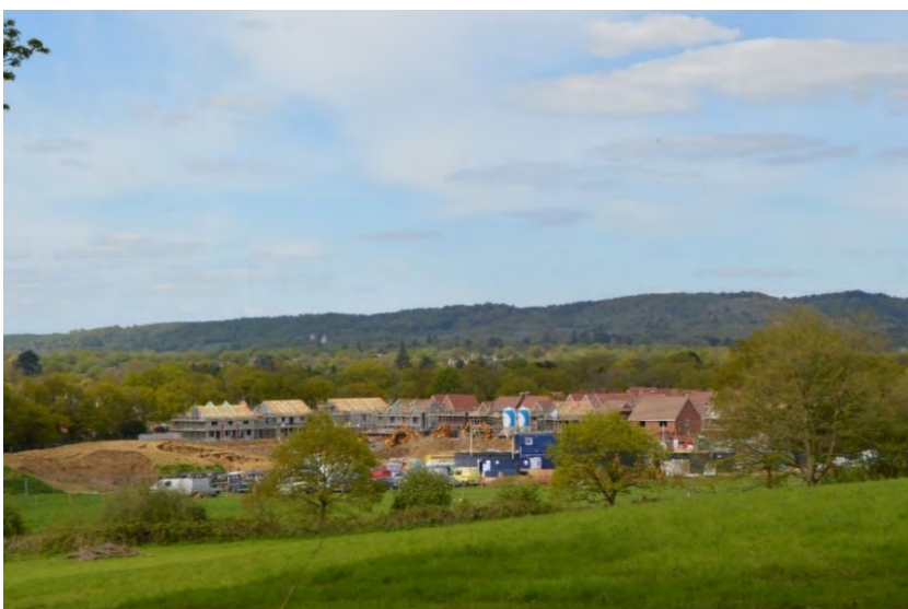
Figure 10: Phase One of development site at Horsham Road under construction
